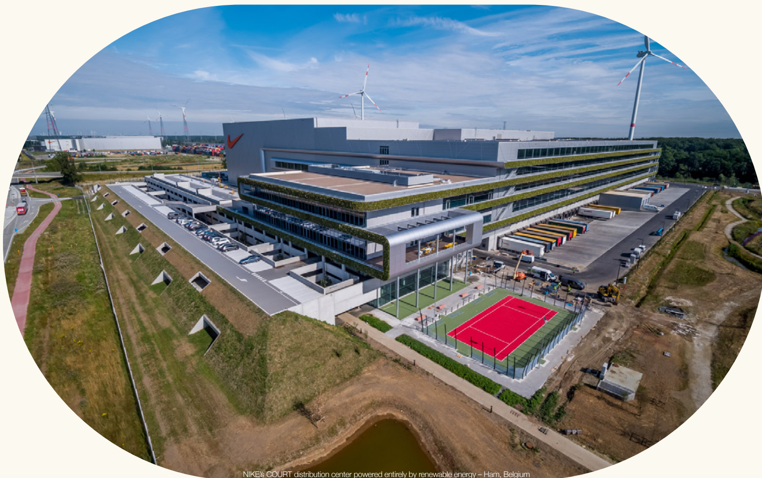
NIKE's COURT distribution center powered entirely by renewable energy – Ham, Belgium
