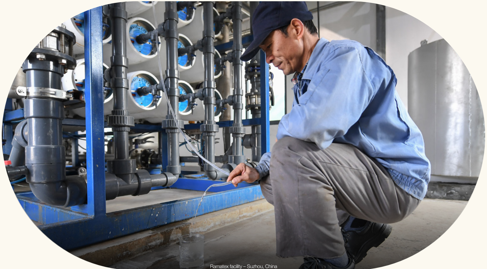
Ramatex facility – Suzhou, China
