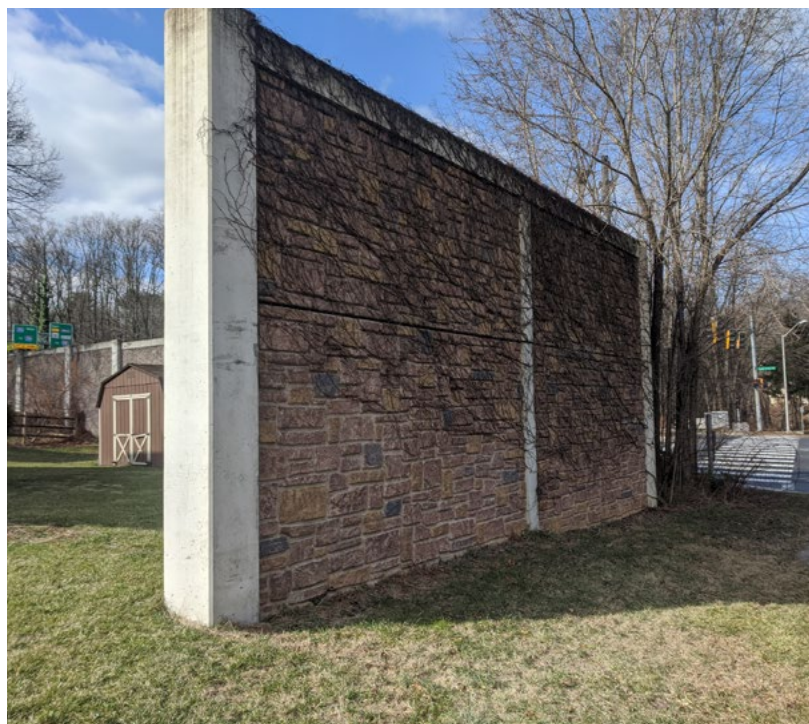
Existing Noise Wall along Shady Grove Road
