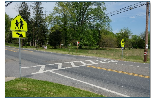
Crosswalk to bus stop at the western end of the high school. This is also marked as an equestrian crossing.
