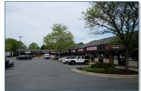
The Ashton Village Center (M-NCPPC Site Plan No. 819841410) was completed in 1986
