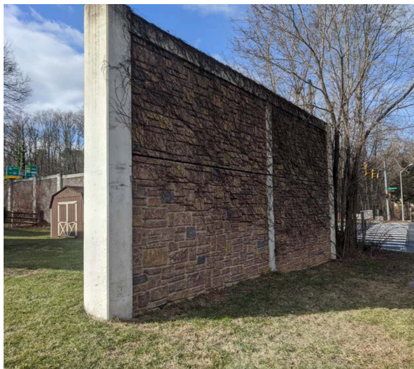
Existing Noise Wall along Shady Grove Road
