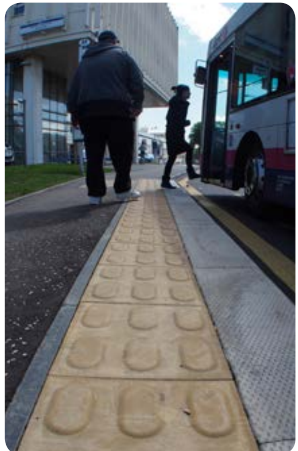
Tactile paving provides distinctive surface patterns to indicate approaching streets and grade changes or mark destinations. Tactile paving should be placed at all bus stops and crosswalks in the study area.
