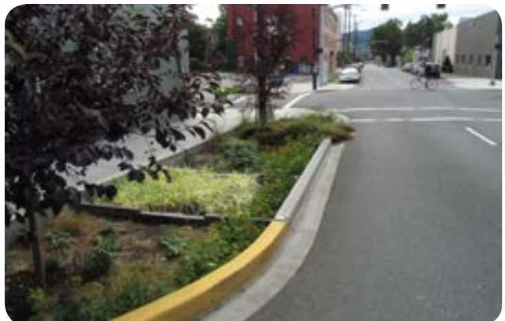
Reflective paint on curbs can help drivers see curb extensions and stormwater facilities along the road, avoiding collisions and damage.
