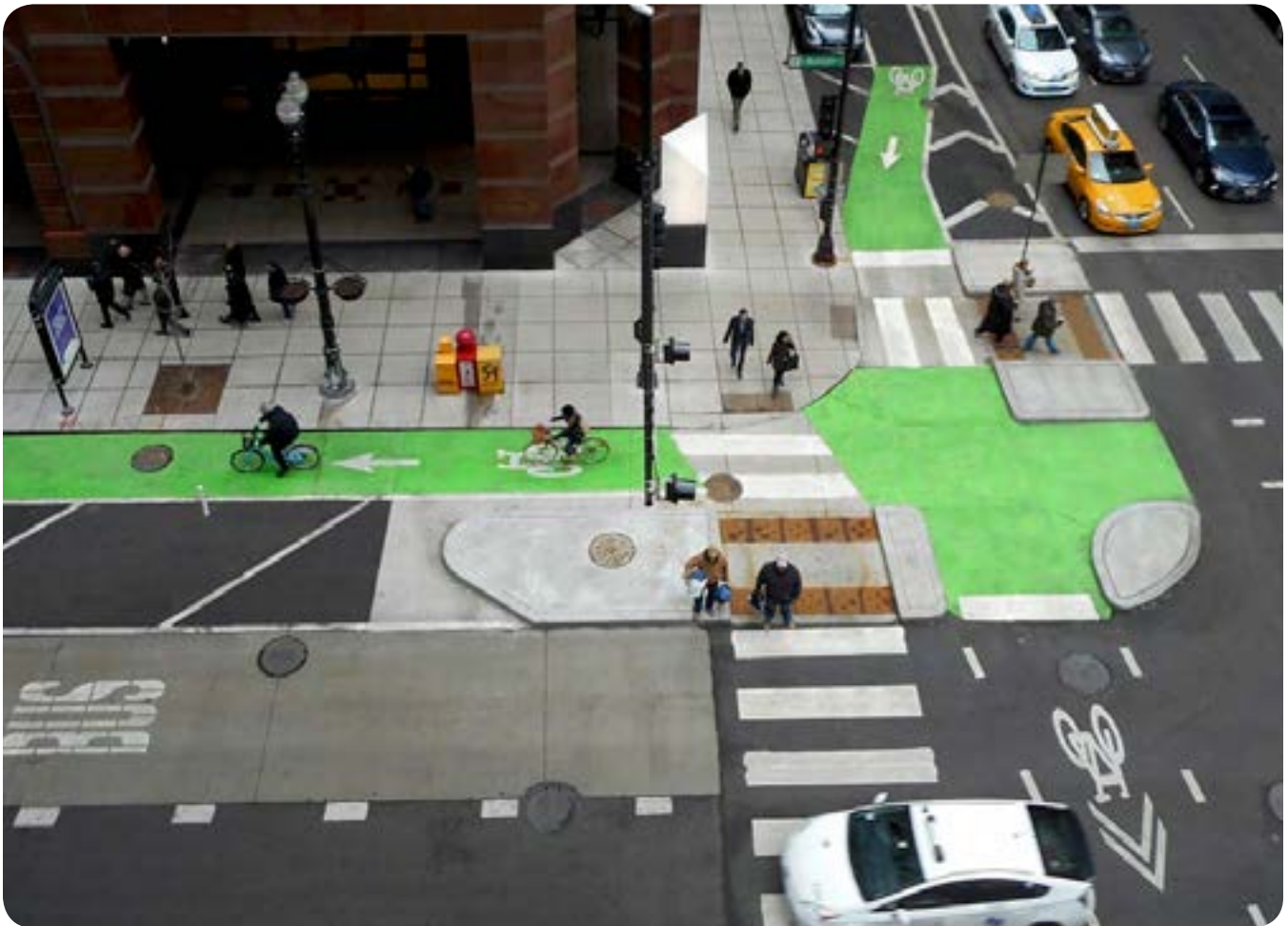
Separate Spaces. Clearly delineated spaces for different road users provide clarity and reduce conflicts. This street provides wide sidewalks, protected bicycle lanes, tactile pavers, high visibility crosswalks, pedestrian islands, as well as signals for people walking, biking and driving.
