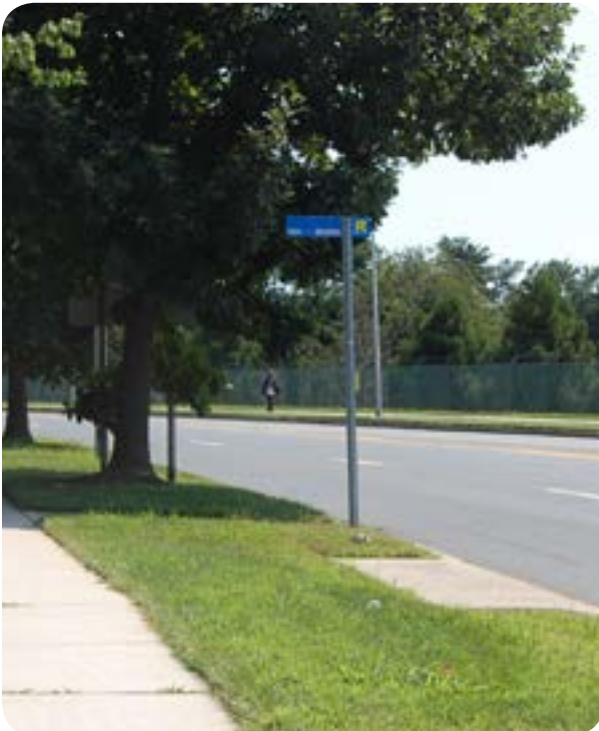
Buffers between the sidewalk and the road, as pictured here on Connecticut Avenue, should be at least five feet wide. Trees planted in the buffer provide additional protection for pedestrians and discourage speeding.
