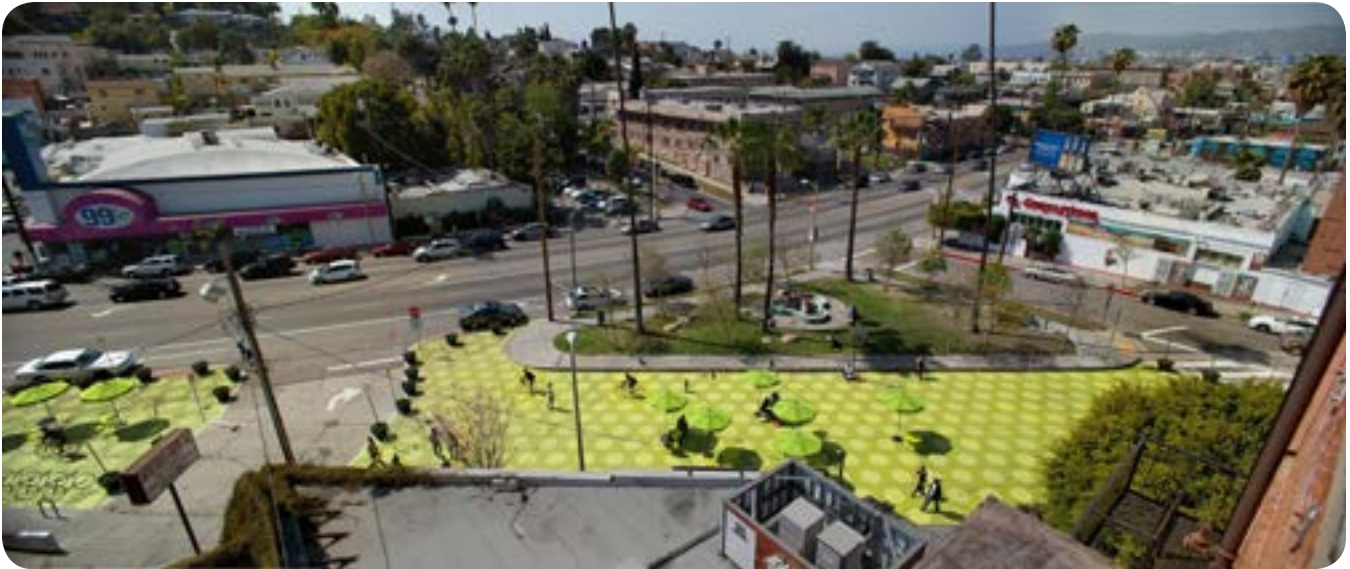
This slip lane in the neighborhood of Silver Lake in Los Angeles was dramatically transformed using only planters and paint. The space reclaimed from slip lanes can provide space for parklets, bike infrastructure, stormwater management, buffers, and wider sidewalks.
